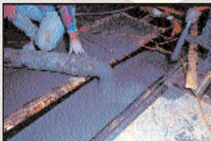
Pumpable castable application
